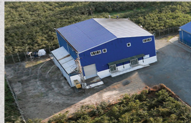
Hazelnut Butter and Hazelnut Croquant Production Facility
