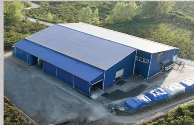
Dry and Cold Storage Warehouse
